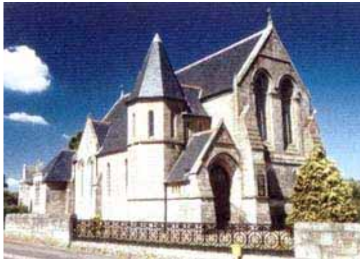
The Quarter Parish Church rebuilt after the fire of 1982.
